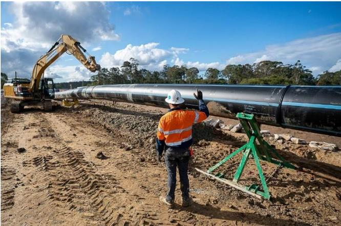
Once the pipe has been unloaded along the construction corridor, the pipes are joined by a welding process. This involves clamping the ends of the pipe together then applying high temperature hot steel plates to melt the two ends of the pipe bonding them and creating a high strength butt weld. The water pipeline is then fully buried, by excavating a trench 1.6 metres wide and up to 4 metres deep in some locations.
