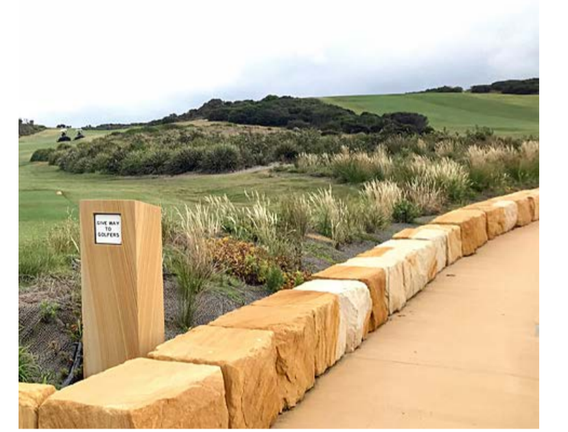
SANDSTONE LOG RETAINING WALL TO PATH EDGE
