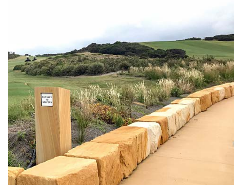
SANDSTONE LOG RETAINING WALL
