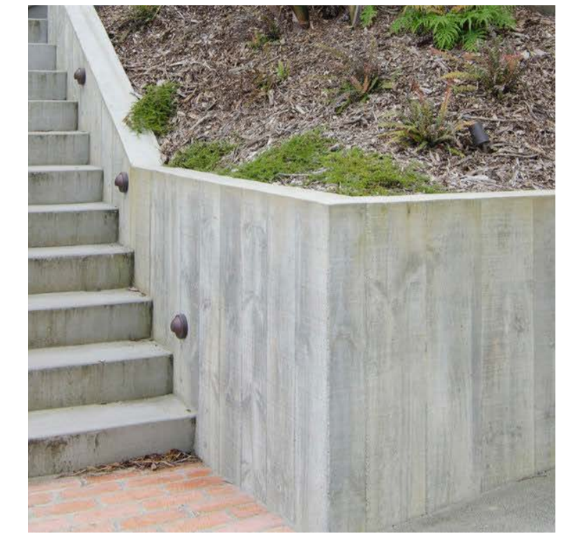
INSITU CONCRETE RETAINING WALL
