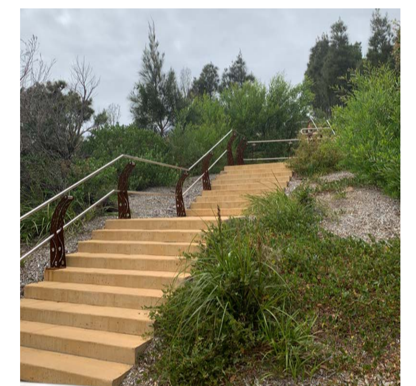
COLOURED CONCRETE STAIRS AND WALKWAY
