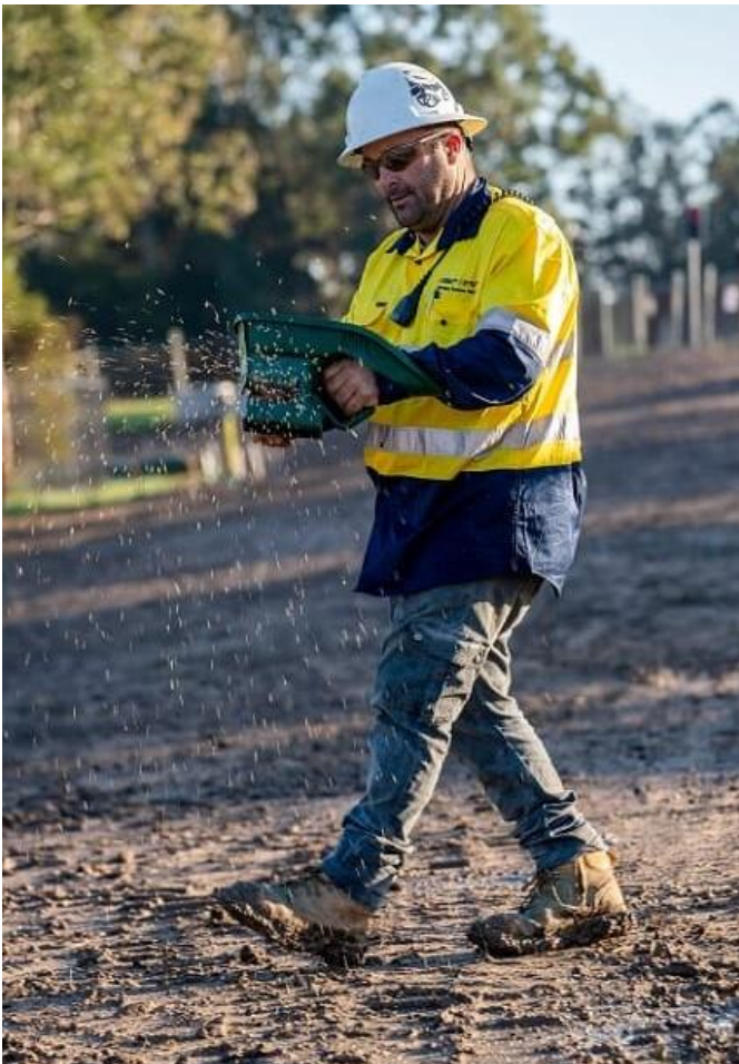
Image: Reinstatement of completed corridor sections with pasture seed
