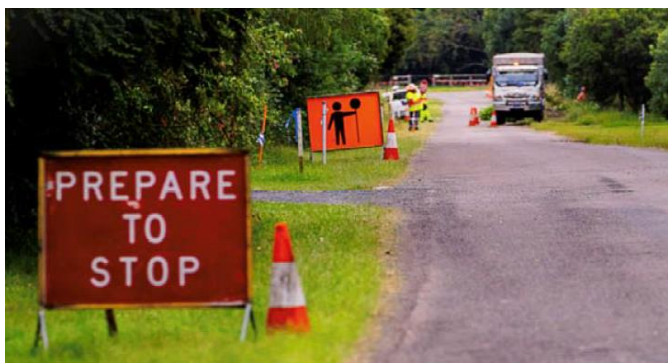
Image: Traffic management keeping the community safe during construction
