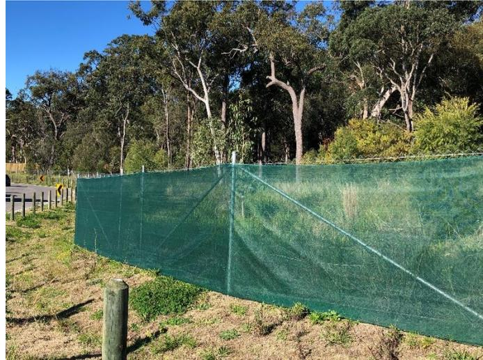
The existing 1.8 metre chain wire fencing with green mesh will be removed from the front of the playspace and replaced with 1.2m high playground fencing to separate the playspace and traffic travelling along Peninsular Drive.
