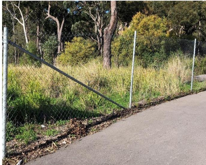
The southern boundary of the playspace will be fenced using 1.8 metre chain wire fencing to deter public access into the protected areas. Fencing will connect to existing fencing along the eastern side of Fairwater Drive.
