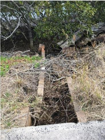
**Figure 18: Man-made drainage channel discharging straight into mangroves; looking west**
